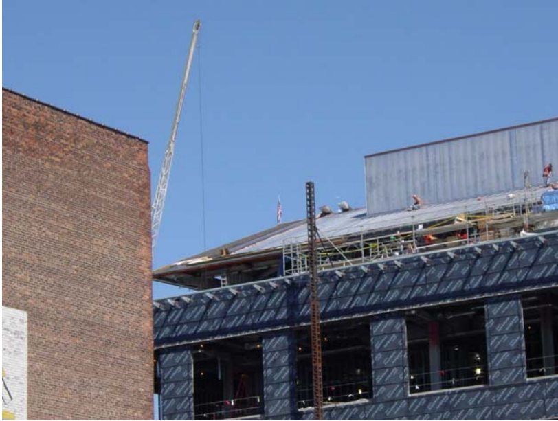
Figure 5. Air barrier on wall at roof edge, extends under cornice.
