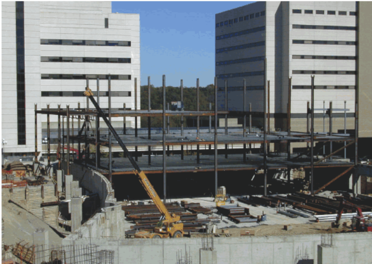
Photos: Douglas Steel Fabricating Corp.
