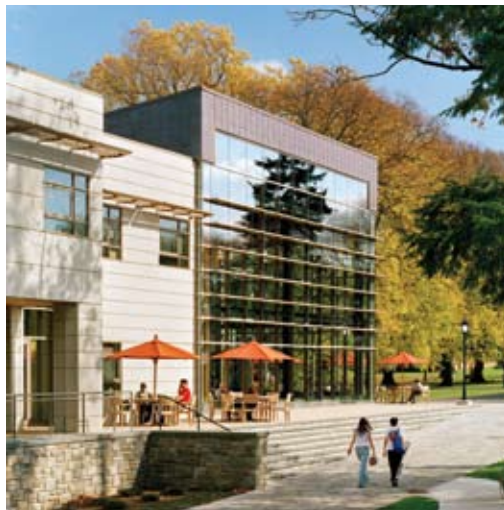
In addition to addressing the impact of runoff, the storm water management system at Philadelphia University's Kanbar Campus Center embodies the concept of "campus as a classroom" for environmental studies.
