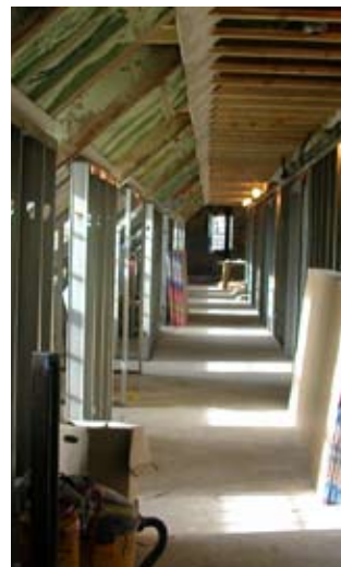
Hallway construction framing
