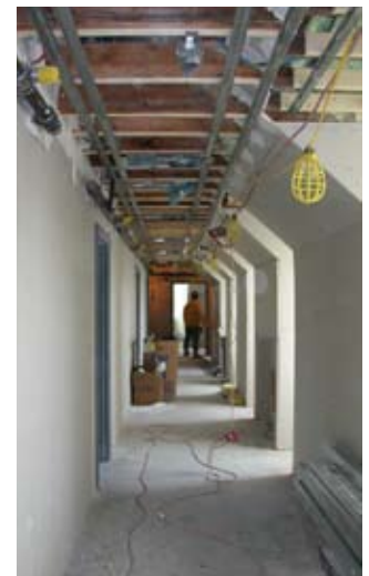
Hallway construction finishing
